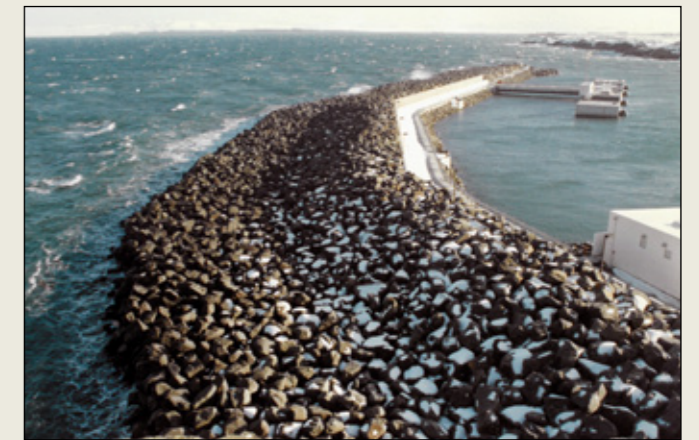
Figure 1.2. Berm breakwater of Helgusvík, Iceland. Designed in 1983 by Baird & Associates and constructed in 1986-1988 by Icelandic contractors.
