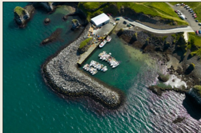
Figure 1.7. The berm breakwater at Arnarstapi, Iceland, sheltering a small fishing harbour. Photo Mats Wibe Lund.
