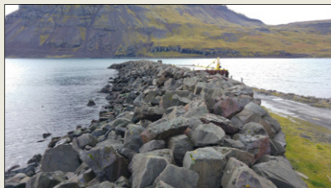
Figure 1.8. The berm breakwater at Nordurfjörður, Iceland, 30 years after construction (1984-1985). Photo R. Kamska.
