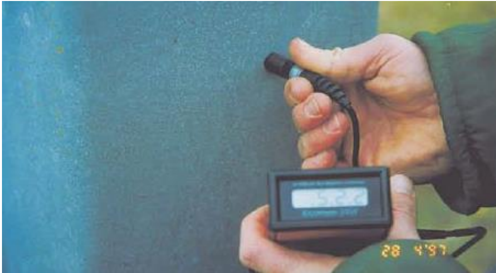
FIGURE 1-1 - MEASURING OF STEEL STRUCTURE THICKNESS [4].
