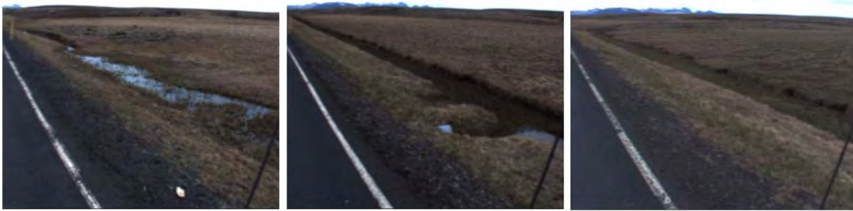
Figure 37: Water standing in the ditches in section 08 but the road is on high embankment, chainage from left to right: 650m, 1120m and 1410m.
