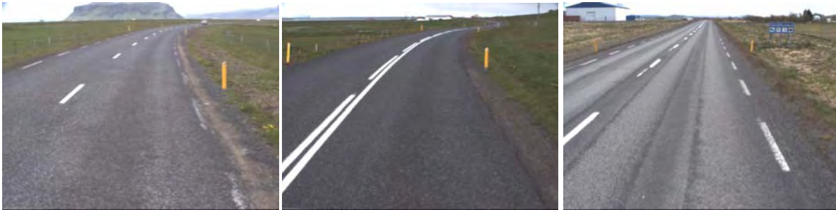
Figure 7: Examples of road sections with drainage Class 2 in Icelandic road network.
