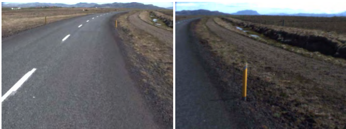
Figures 27: Water standing in the ditch behind the horse track, chainage 6300m-6500m.
