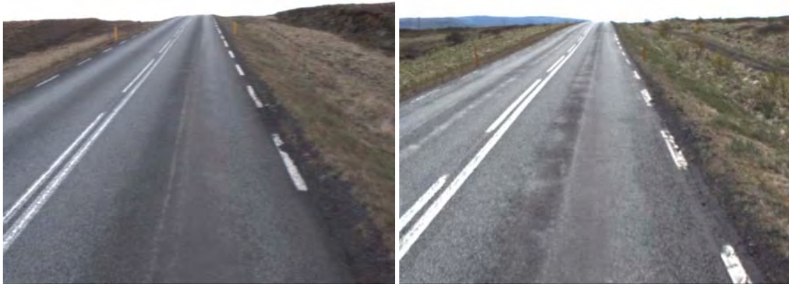
Figure 41: Examples of verge, chainage 8450m (left) and 10640m (right).
