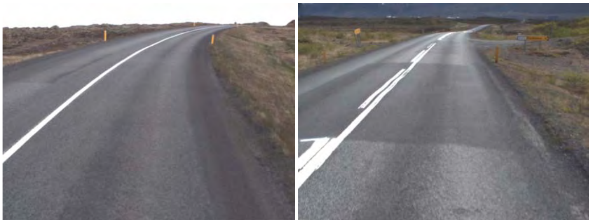
Figure 50: Example figures of verge at chainage 1270m and 2690m.
