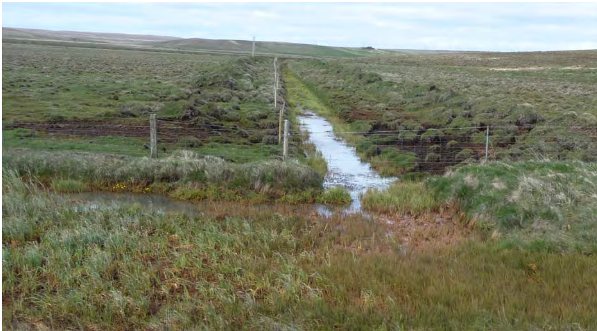
Figure 26: Outlet ditch full of vegetation and water, chainage 2730m.
