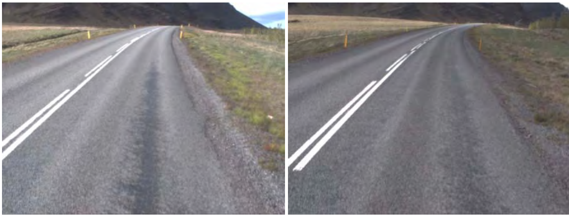
Figure 49: Minor verge at chainages 10220m and 10340m.
