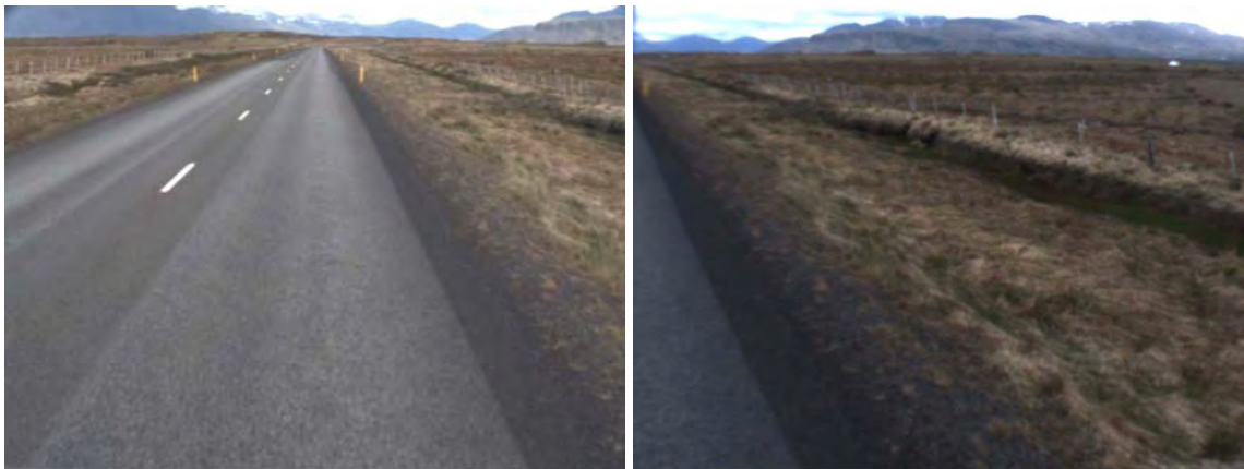
Figures 54: Water and vegetation in the ditch, chainage 1740m. The left figure is the road camera view and the right figure is the ditch camera view.
