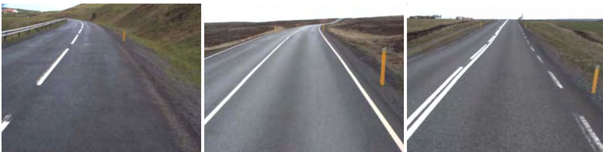
Figure 6: Examples of road sections with drainage Class 1 in Icelandic road network.
