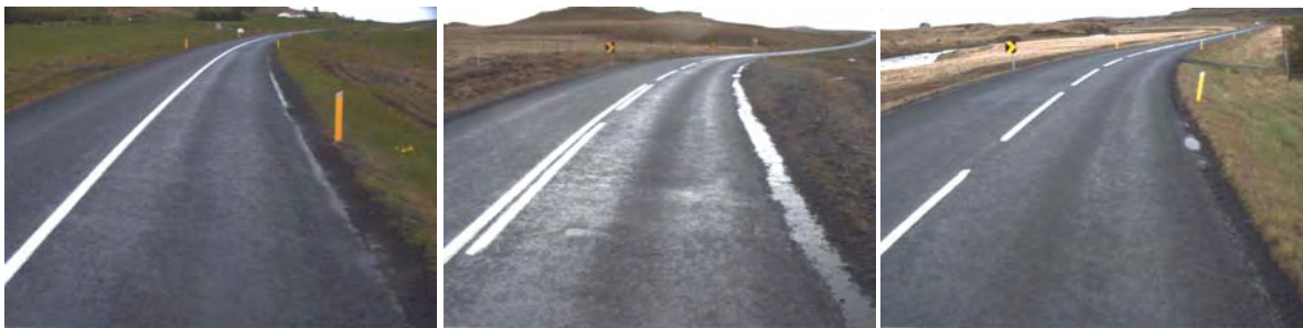
Figure 10: Examples of verge Class 2, roads with a verge. The effect of verges on the workings of the road drainage system varies greatly in different circumstances.
