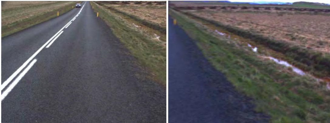
Figure 31: Water stays in the ditch on the left side, left figure is the road camera view and the right figure is the ditch camera view (chainage 1090m from direction 2).
