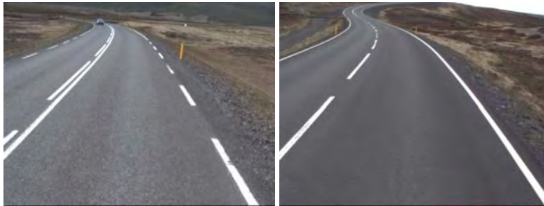
Figure 9: Two examples of verge Class 1, i.e. road sections without verges.
