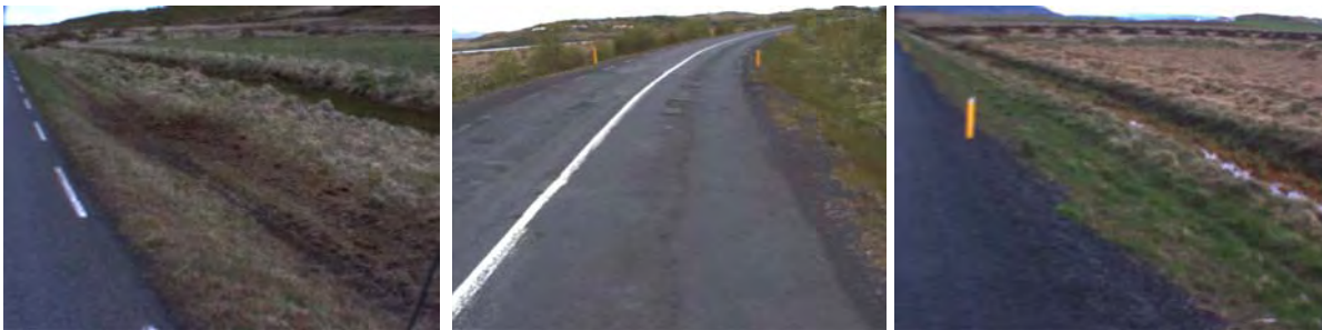
Figure 8: Examples of road sections with drainage Class 3 in Icelandic road network.
