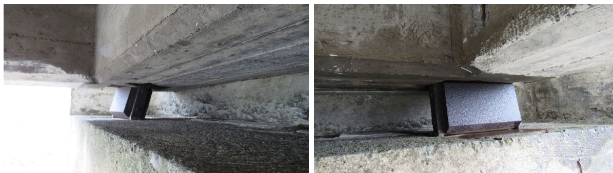
Figure 4.4: Photos of the end support rollers (photo Einar Óskarsson, IRCA).
