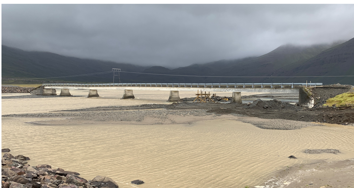
Figure 1.2: The Steinavötn bridge in August 2019, view from southeast.
