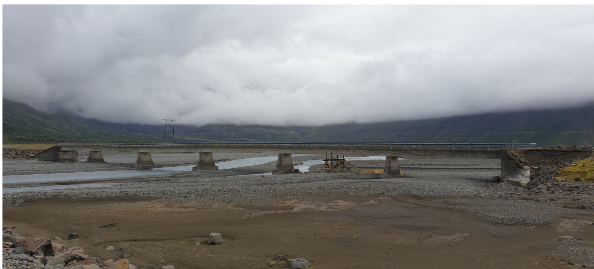
Figure 1.1: The Steinavötn bridge in July 2019, view from southeast.
