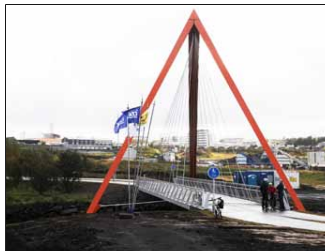
Pedestrian bridges over Elliðaár
